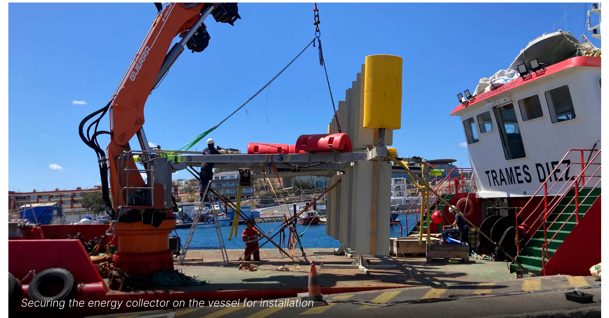
Full-scale energy collector being installed at PLOCAN, Gran Canaria
